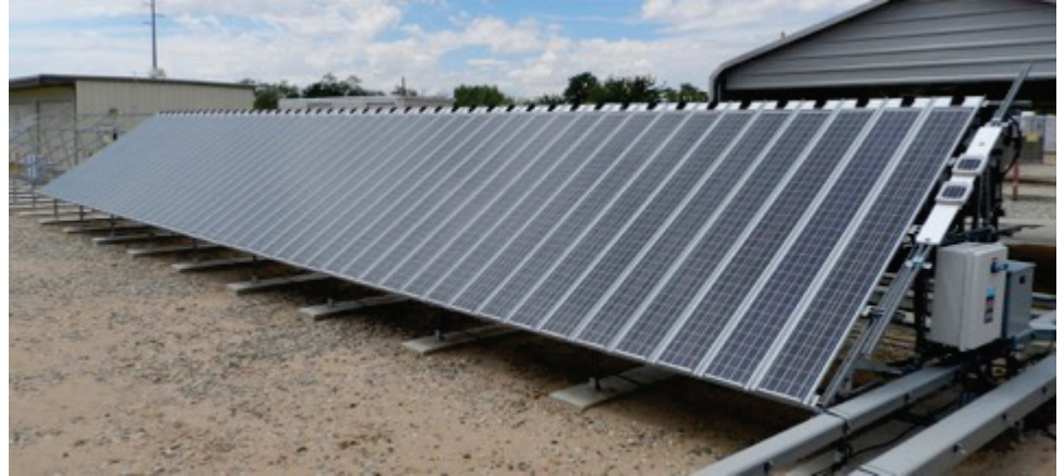
System Level: Prototype flexible CIG modules installed on roof pans
