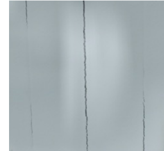
PA Backsheet cracking
