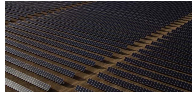
A large-scale solar farm
