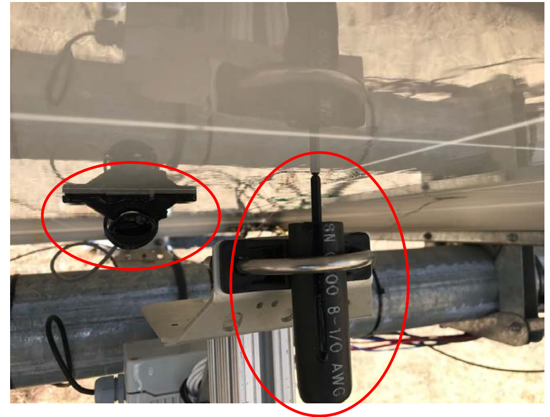
Potentiometer to measure displacement and accelerometer to measure vibration
