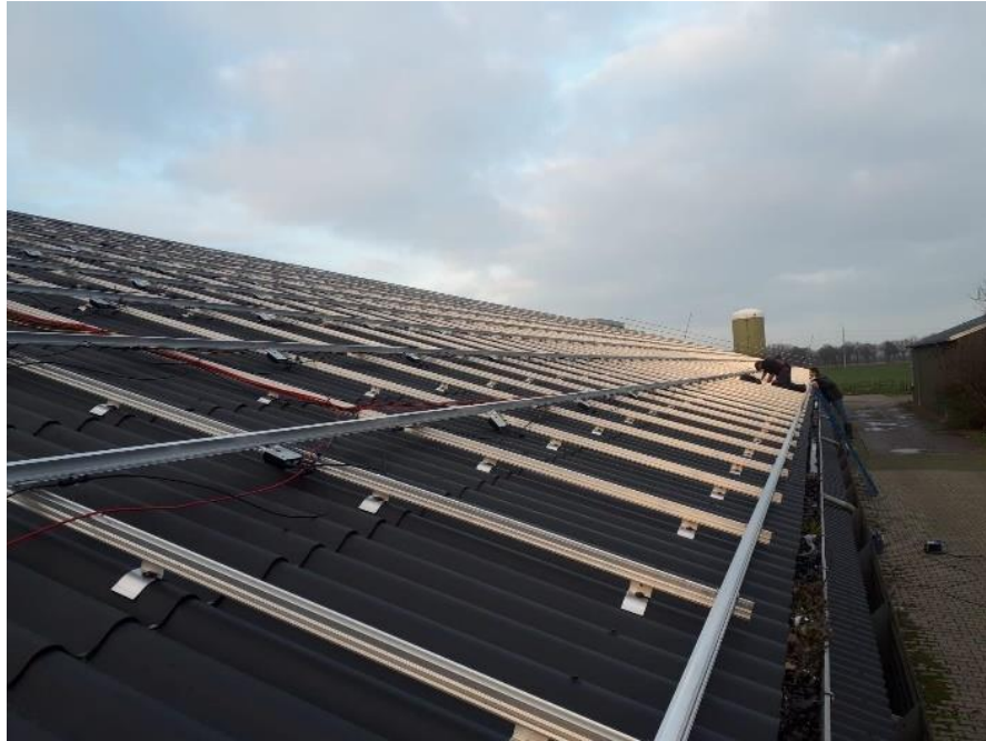
Mounting system for corrugated rooftiles
